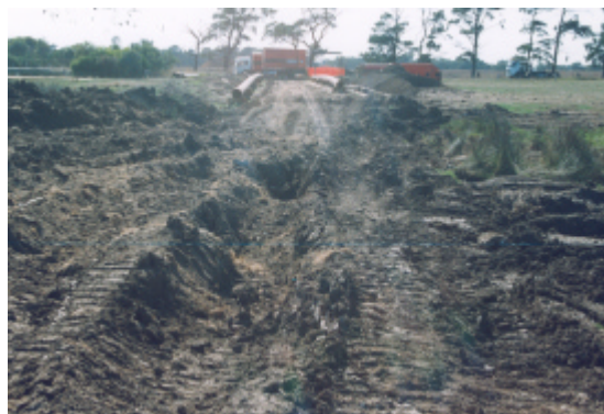
Typical result of traffic on this soil type
